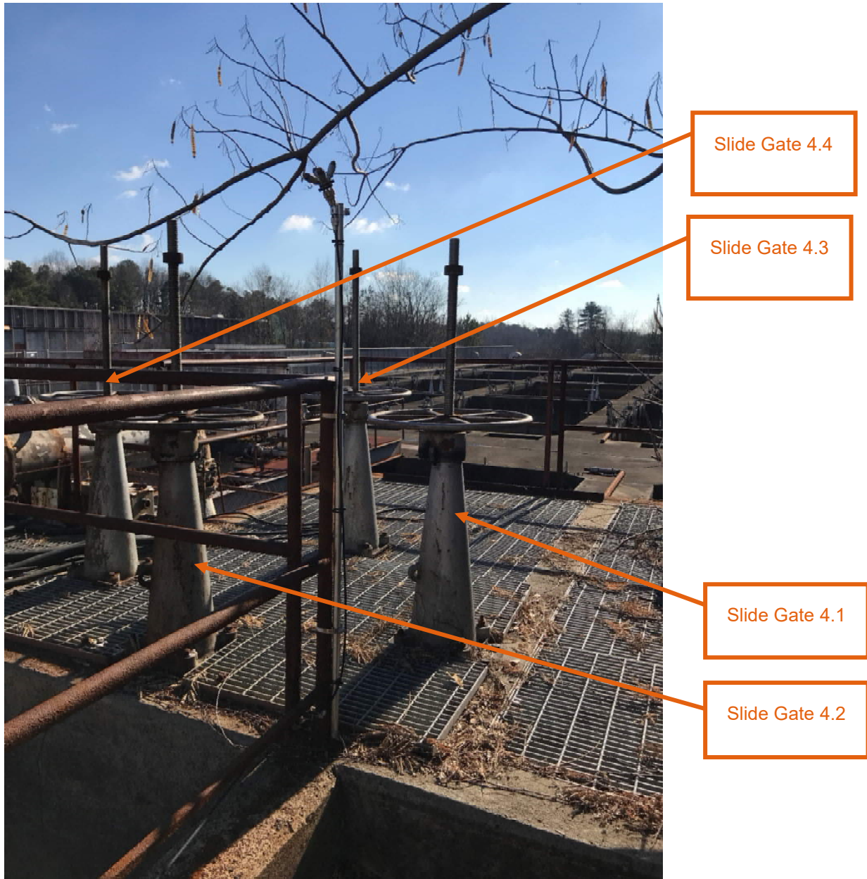
Figure 33: Overflow Weir Slide Gates 4.1, 4.2, 4.3, and 4.4
