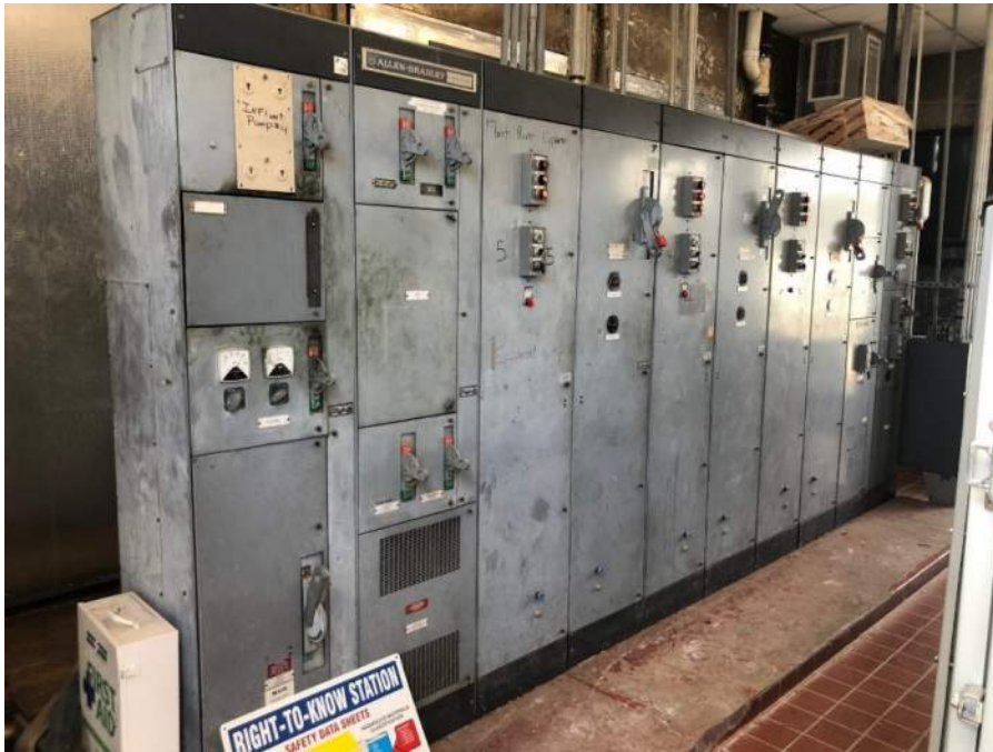
Figure 14: Motor Control Center (MCC)
