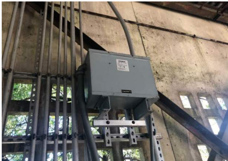
Figure 25: Transformer TA Junction Box
