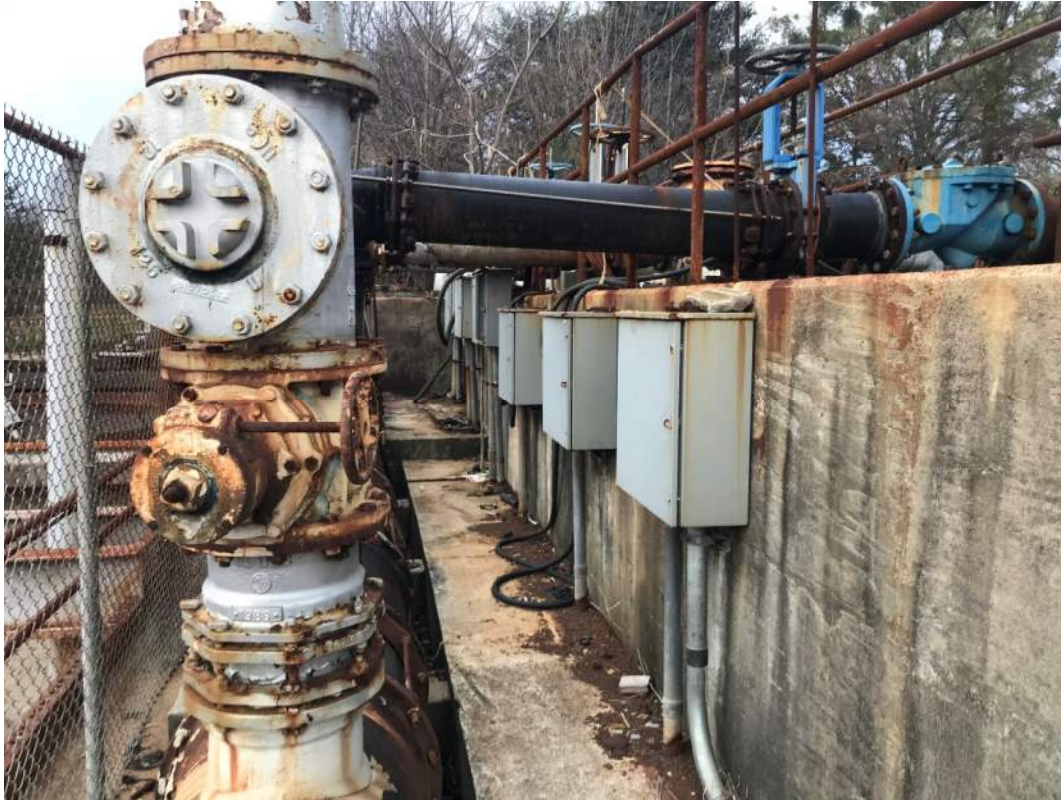
Figure 34: Effluent Pumps Cable Junction Boxes
