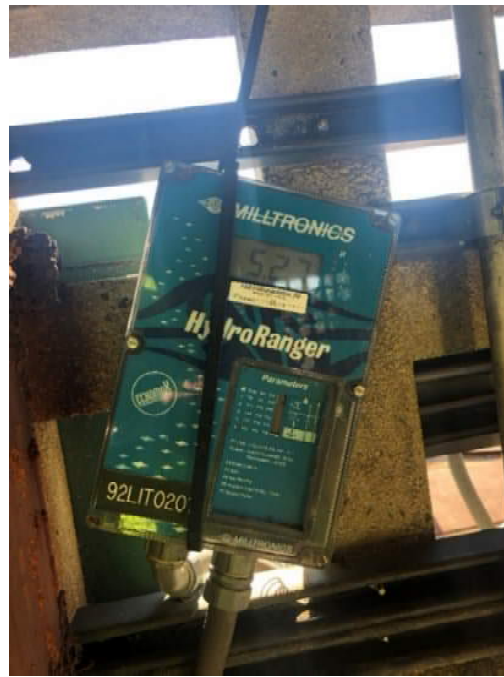
Figure 26: East Flume 3.1 and West Flume 3.2 Level Sensor Controllers
