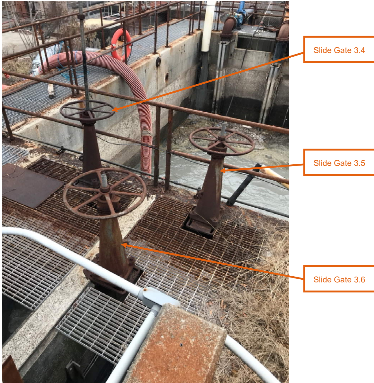
Figure 22: Flume Effluent Slide Gates 3.4, 3.5 and 3.6
