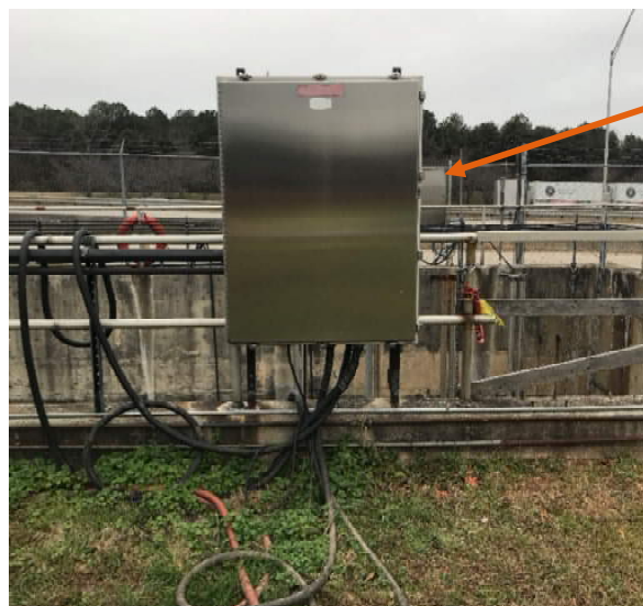
Figure 8: Pump 1.4 and 1.5 Local Disconnect
