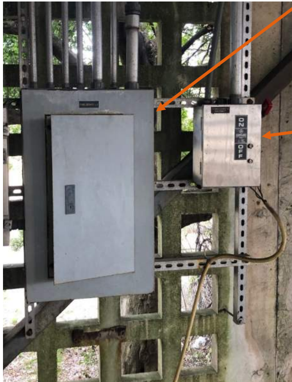
Figure 24: Panelboard LA and Transformer Disconnect Switch
