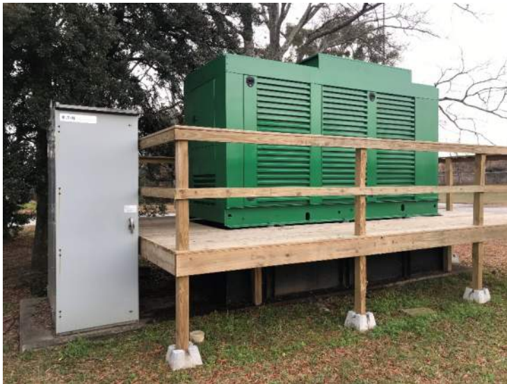
Figure 13: Switchgear and Diesel Generator
