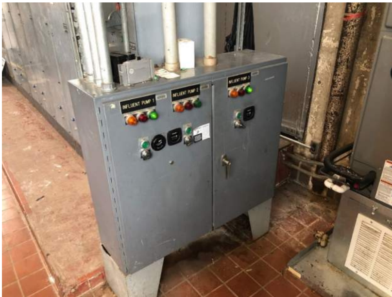
Figure 15: Pump 1.3 and 1.4 Control Panel
