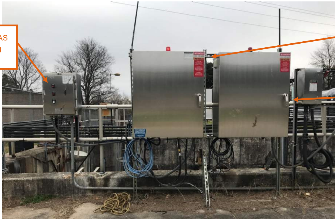
Figure 7: Flygt Local Control Panels
