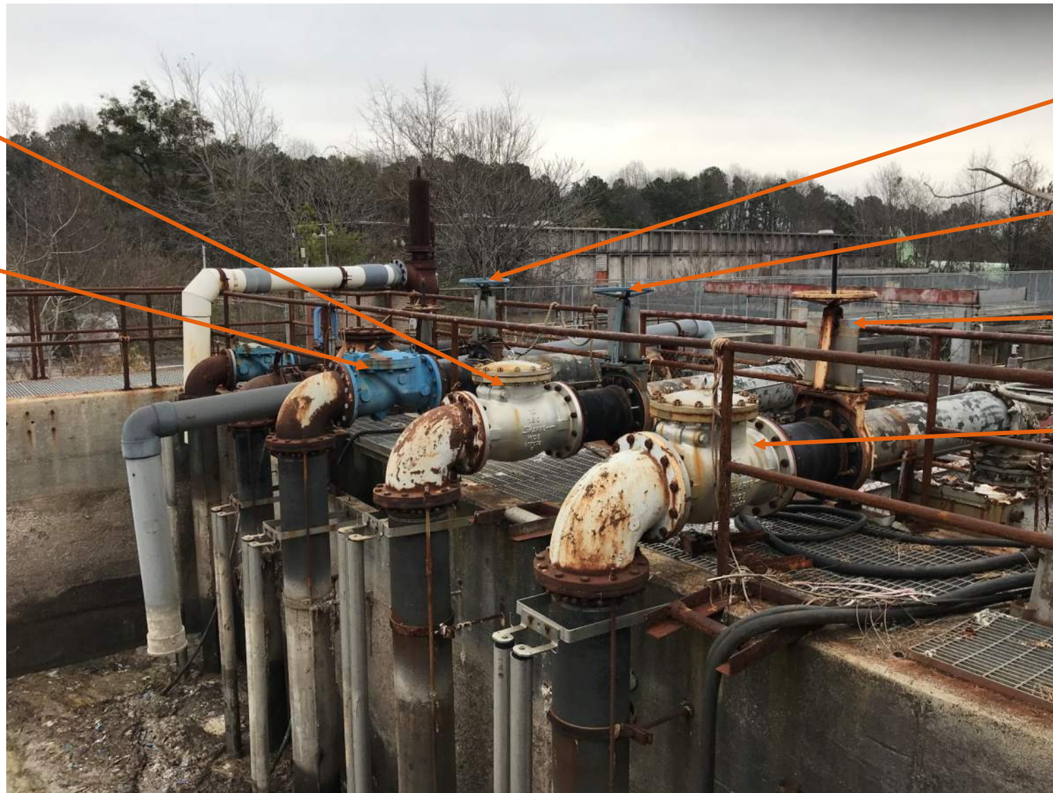
Figure 31: Pumps 4.3, 4.4, and 4.5 Discharge Piping
