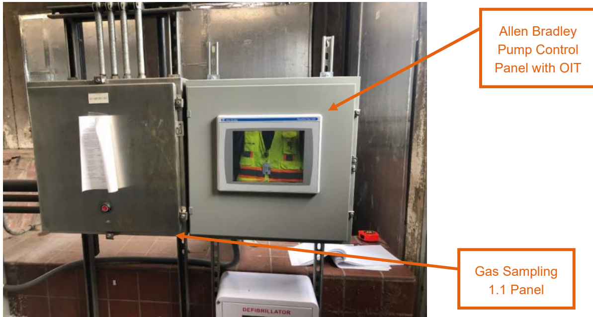
Figure 18: Gas Sampling System 1.1 Panel and Allen Bradley Pump Control Panel with OIT
