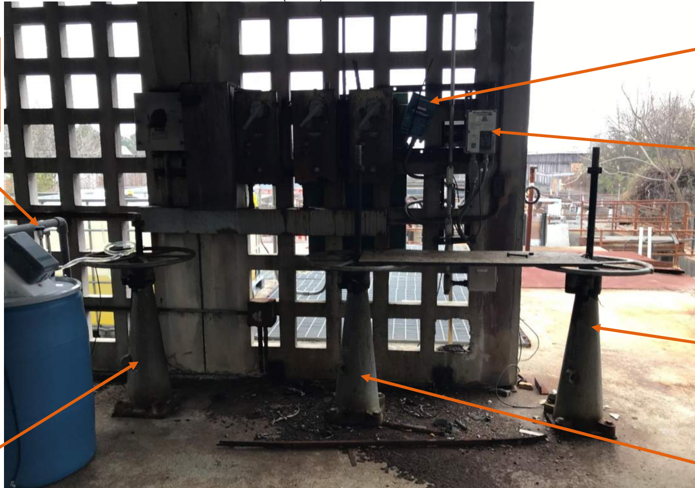
Figure 20: Screening Building Effluent Slide Gates and Flume Level Sensor Controllers
