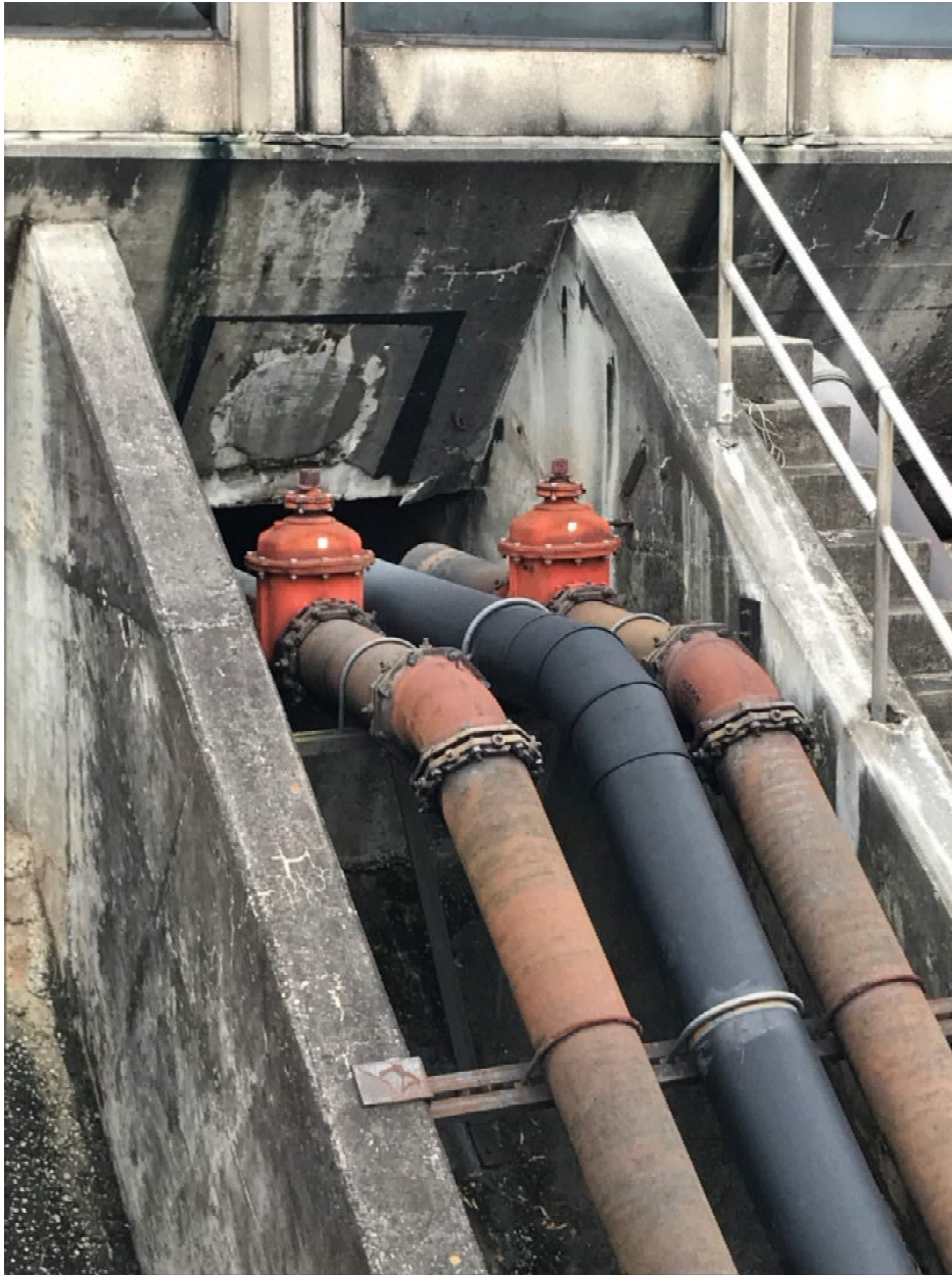
Figure 3: Gate Valve 1.5 and 1.6
