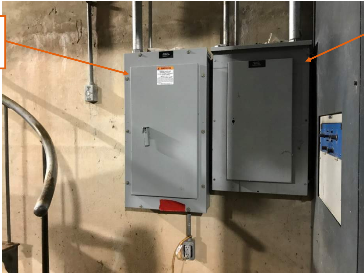
Figure 40: Clarifier Pump and Sump Pump Panels LP-1 and HP-1
