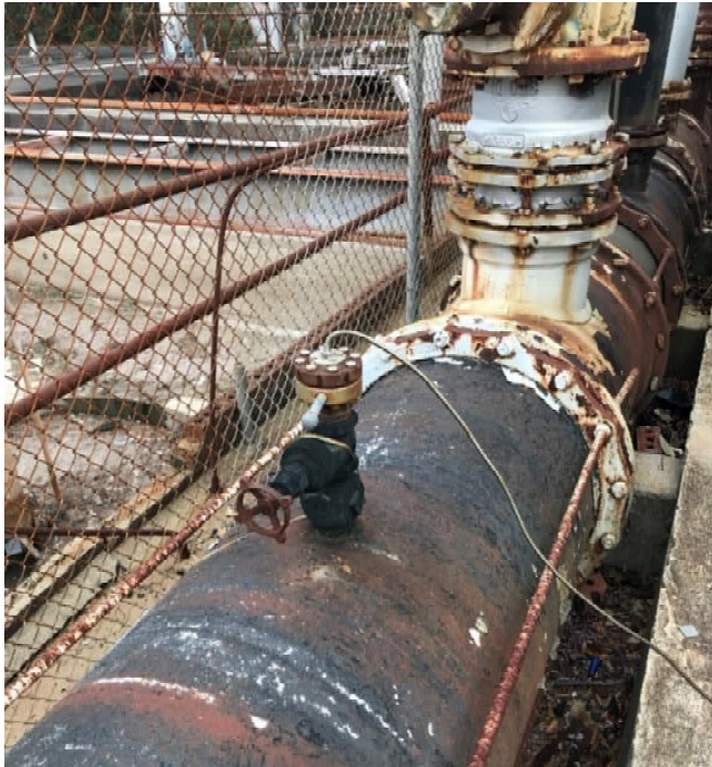
Figure 36: Pressure Sensor 4.1
