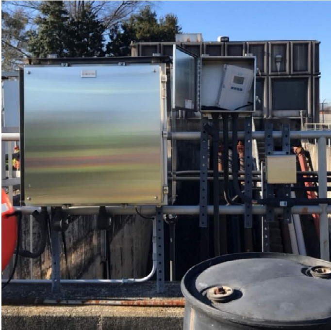
Figure 9: Level Sensor 1.1 Control Panel Exterior and Interior
