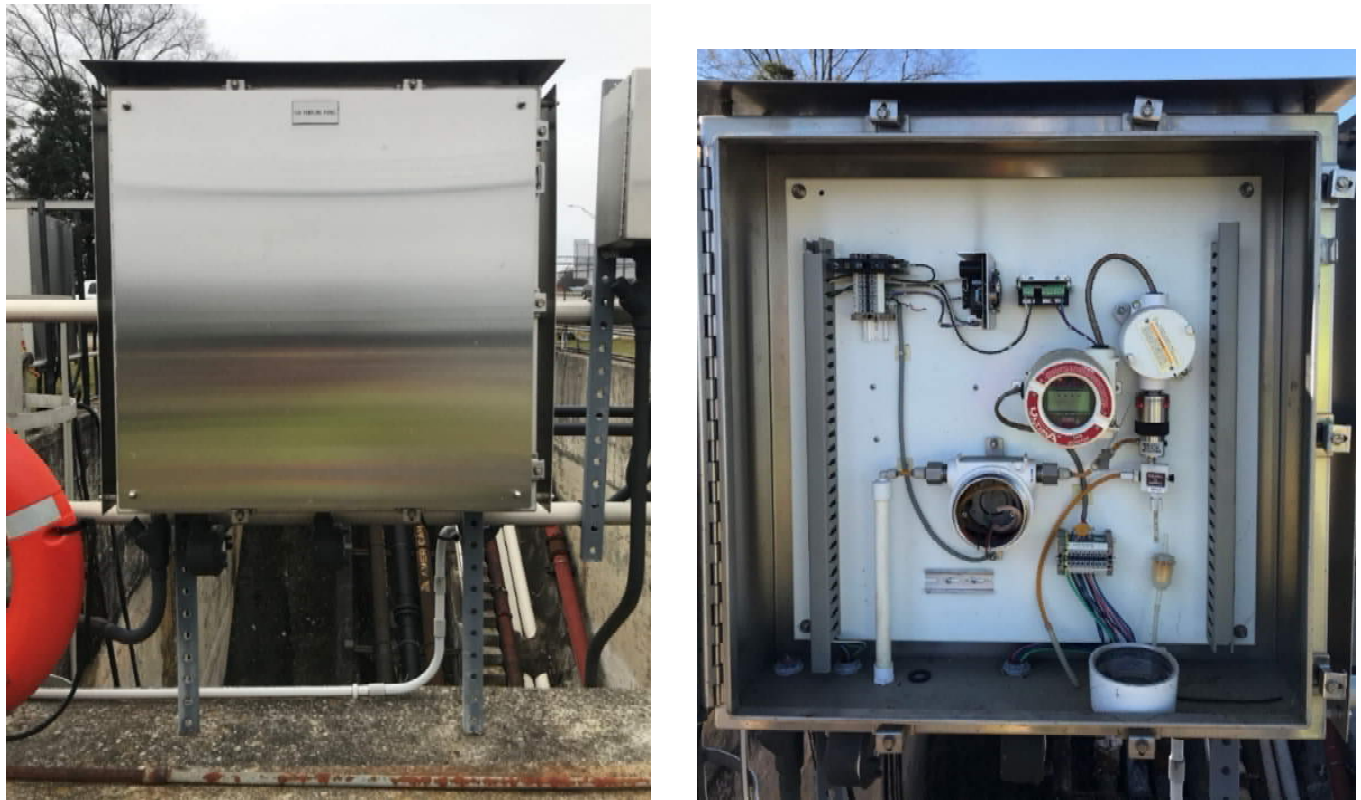
Figure 11: Gas Sampling System 1.1 Panel Exterior and Interior
