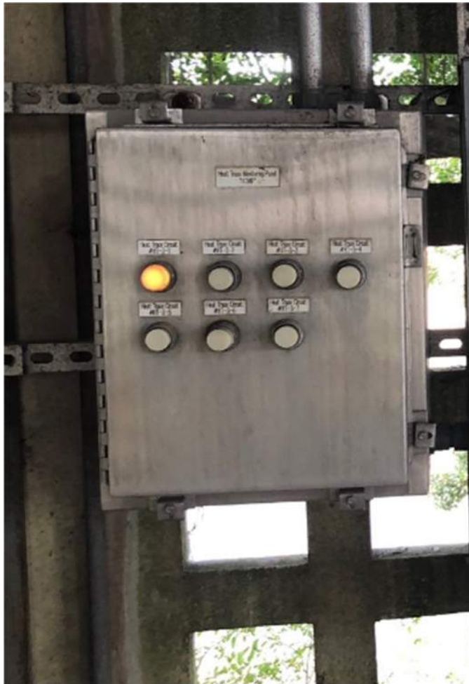
Figure 28: Chemical Heat Trace Monitoring Panel
